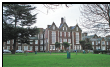
The western elevation of the main administration block, dated 1840, was once the front of the Hospital. Wings were added later on either side.
