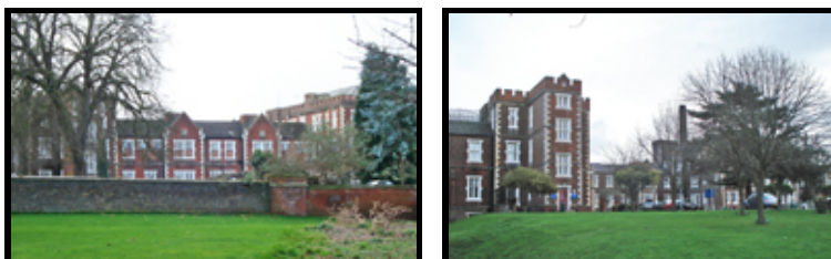
The northwest side of the Hospital (left). The male ward block (right).
