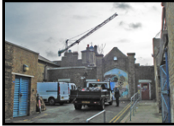
The workshop and utility area of the Hospital in the centre of the site.
