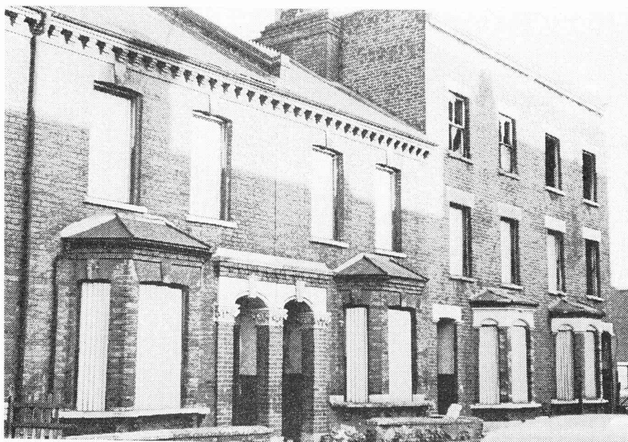
Fig. 5: Houses awaiting demolition in Wickersley Road.
